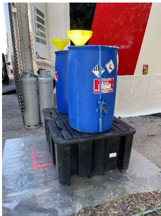
Oil drums are properly secured, and the ground is protected by two layers of spill covers.
